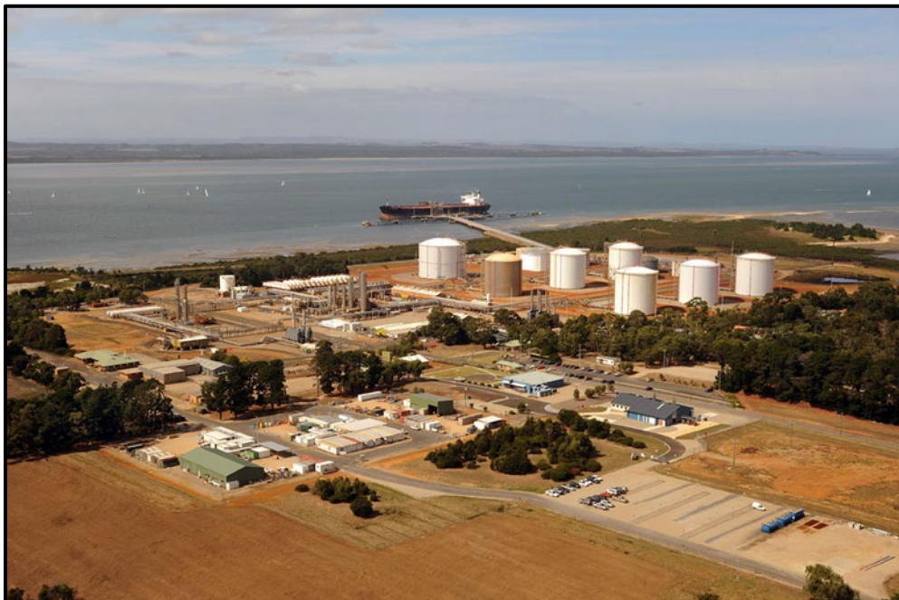
Figure 1 Long Island Point (LIP) LPG Fractionation Plant
