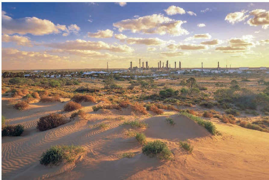
FIG. 1. The Moomba gas plant in South Australia.
