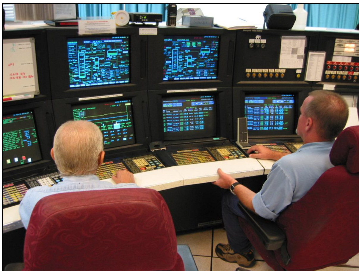
Figure 3 – Panel Operators using the new APC system in Brisbane, Australia.
